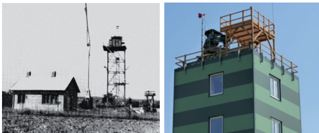
Fig. 2. The initial AUT site of far-field outdoor range (left) and the renewed tower, AUT and vertical positioners.
