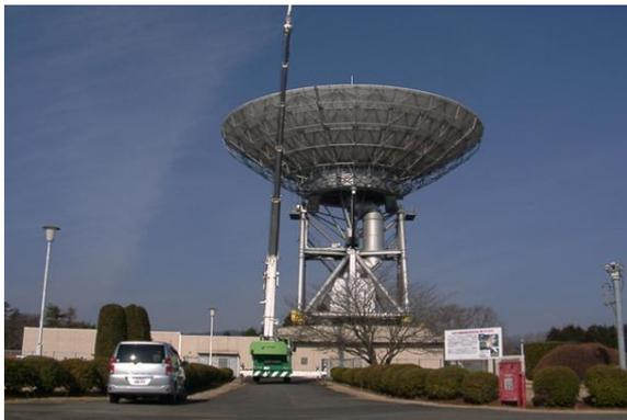
Fig.14. Feed installation.
