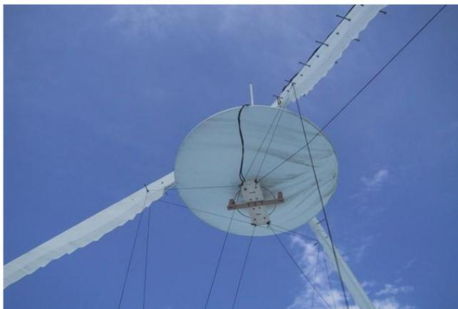
Fig. 15. "Marionette style" tension cable mechanism.
