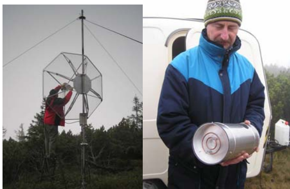
Fig. 13. The loop feed being assembled into the dish.
